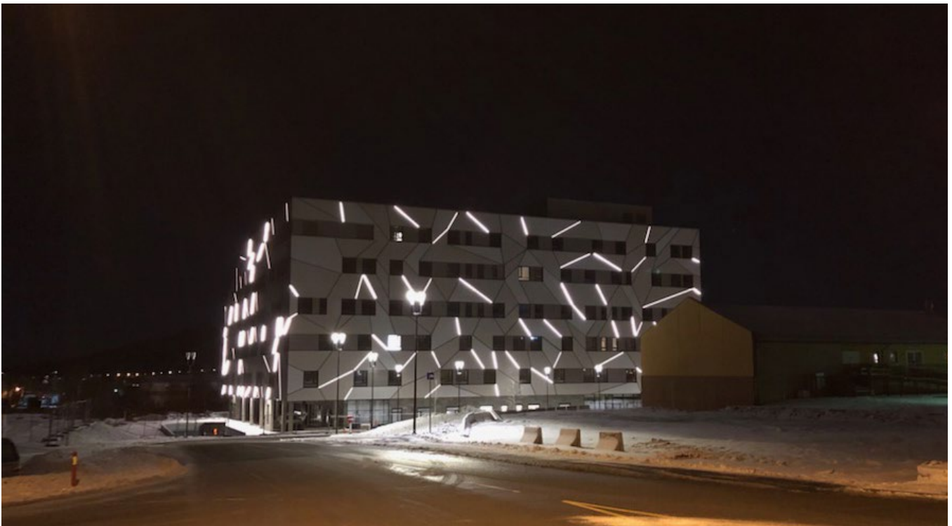
Region Nordhordland Health Center is being built to co-locate health services for the inhabitants. The health center will have a passive house standard, and will be heated using heat pumps, which covers 85% of the annual heat demand. The building is financed with a green loan from KBN. Photo: Altifilm AS
