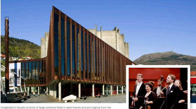
Grieghallen's facade consists of large windows fixed in steel frames and are original from the 1970s. Several of these are cracked or punctured. Both the windows and the steel frames have poor insulating properties. Now all 550 windows will be replaced, and the steel frames insulated. It is estimated that the total energy savings for the project is 1,000,000 kWh/year. Photo: NTB.
